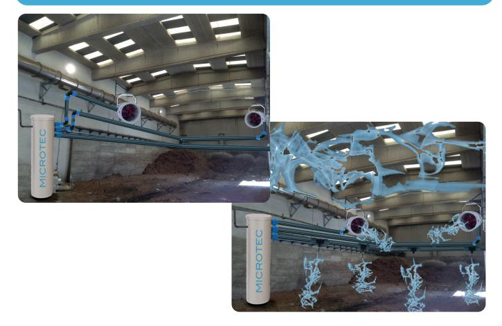
The **MICROTEC** FAN (optional) peripheral device, connected to a **MICROTEC** unit, ensures constant contact between the two gaseous phases by a continuous mixing of the volumes of air to be treated.
